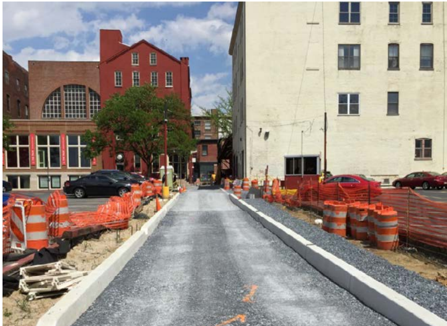
Grant Street Reconstruction
