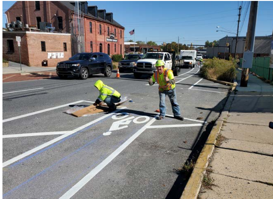
Walnut Street Repainting
